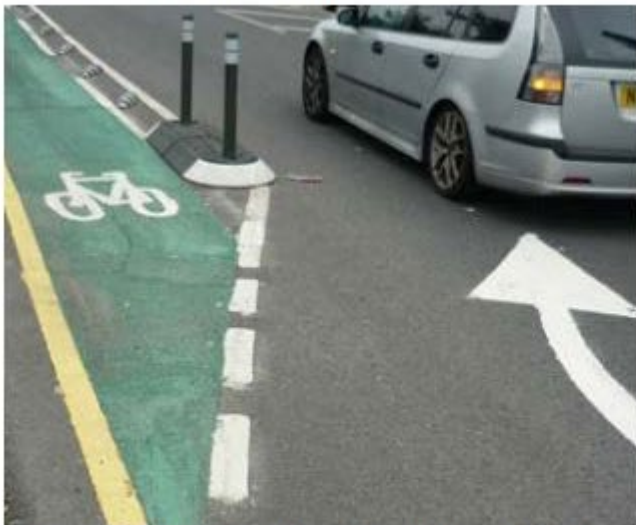
Temporary island at the beginning of a run of separators (Salford trial)
