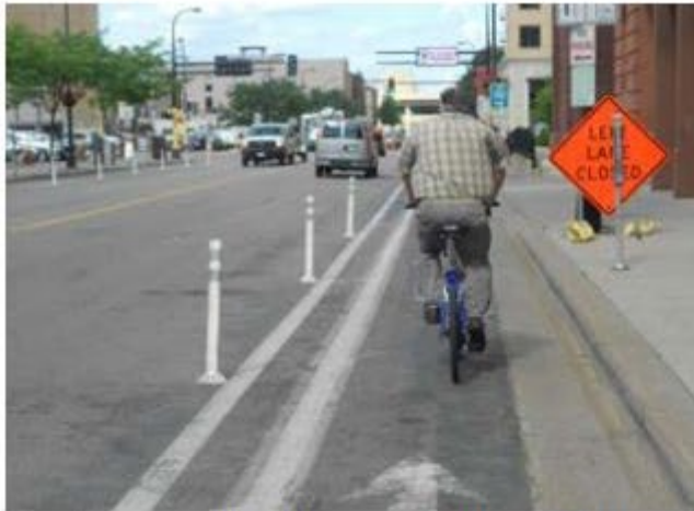
Light segregation with posts in Minneapolis
