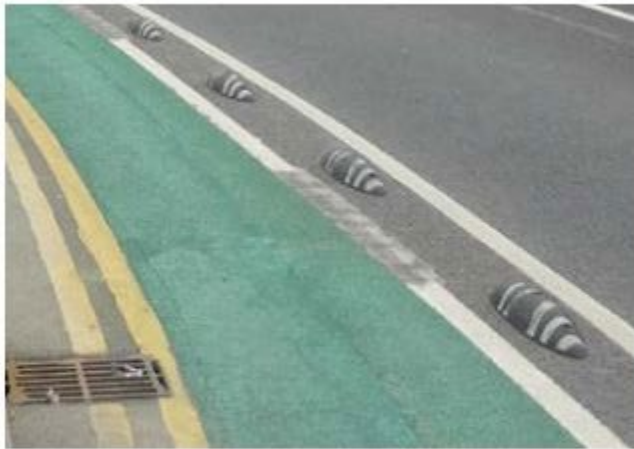
Pre-formed separators used next to cycle lane markings (note that only one lane marking should be used)
