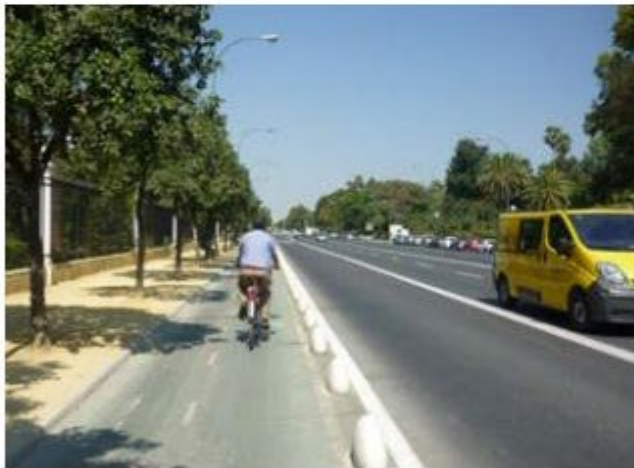
Use of concrete 'lacasitos' in Seville
